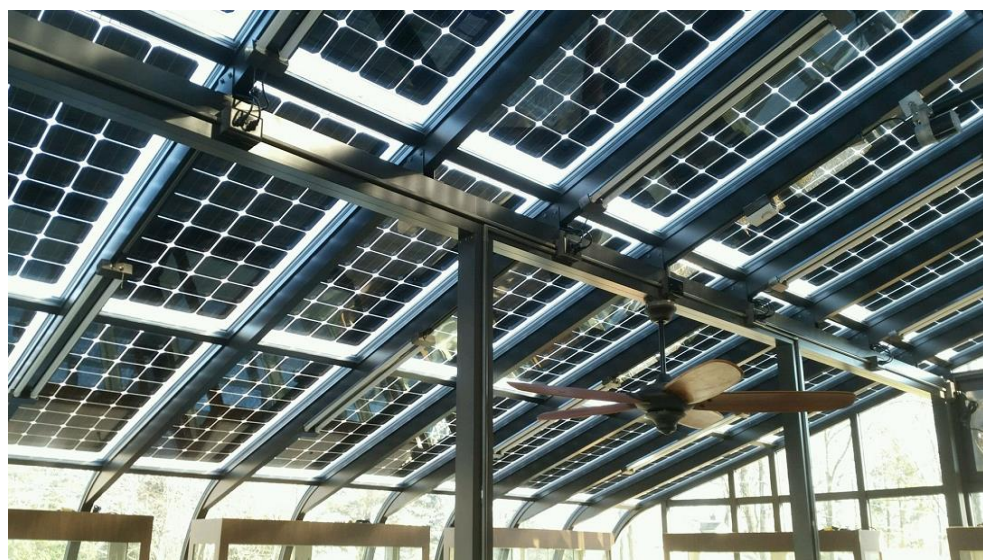
Traditional Double Glass Solar Rooftop: Bulky system with comprehensive supporting metal structures. Low solar-to-roof space utilization.
