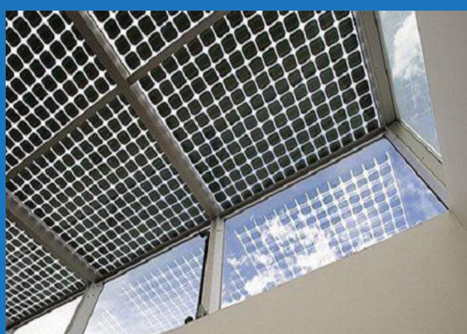
BIPV Transparent Double Glass Solar Rooftop
